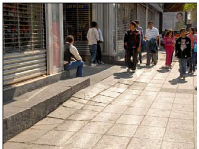
The subsided and distorted street pavement alongside the relatively stable Torre Latinoamericana.
