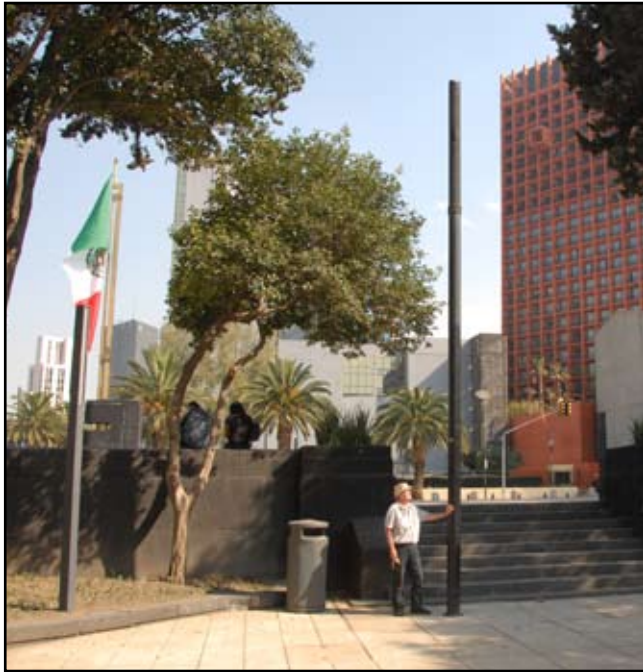
The protruding well casing in Plaza de la Republica.
